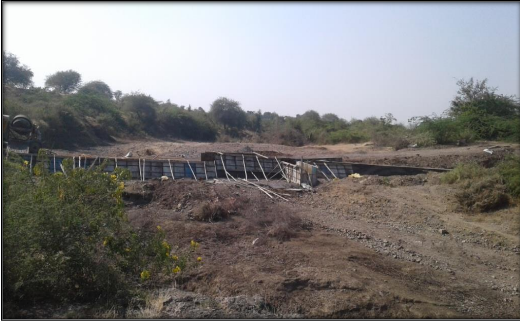
Picture:2 During progress work of Check dam
