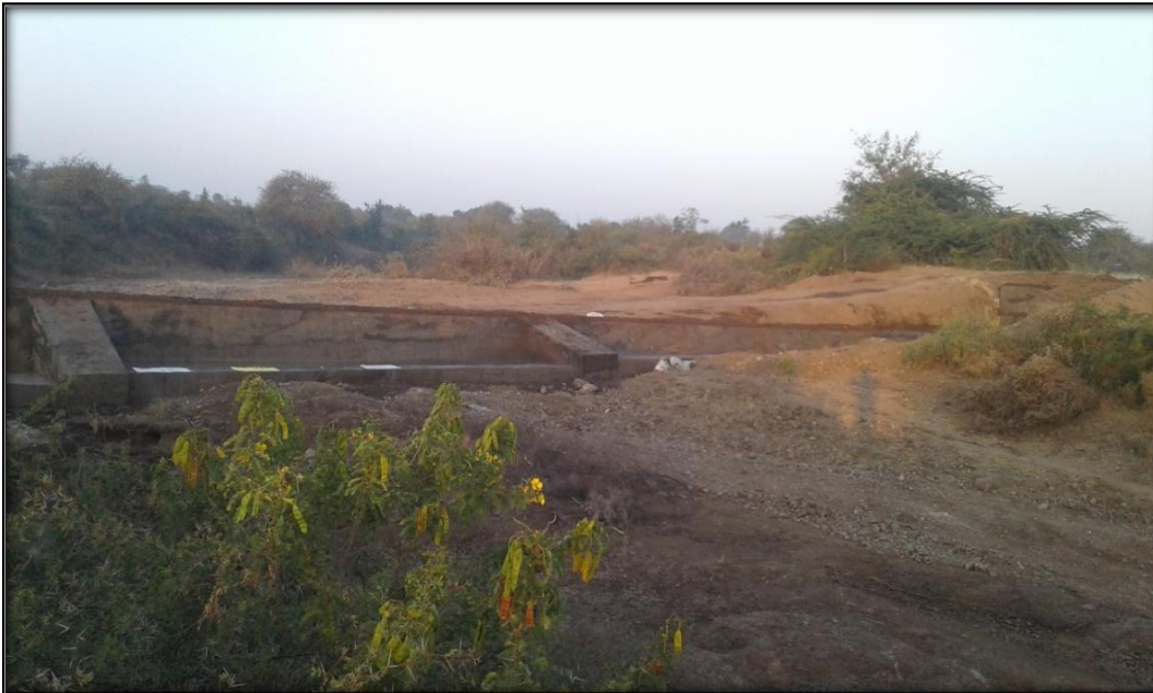
Picture-3 Completed Check dam
